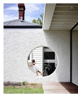
TEXTURED PAINT WALL. TIMBER DECK FOR TERRACE BALCONY WITH EXPRESSED JOISTS
