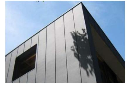
FIBRE CEMENT CLADDING WITH VERTICAL JOINTS AND PAINT FINISH WITH FINE COLORBOND CAPPING TO PARAPET
